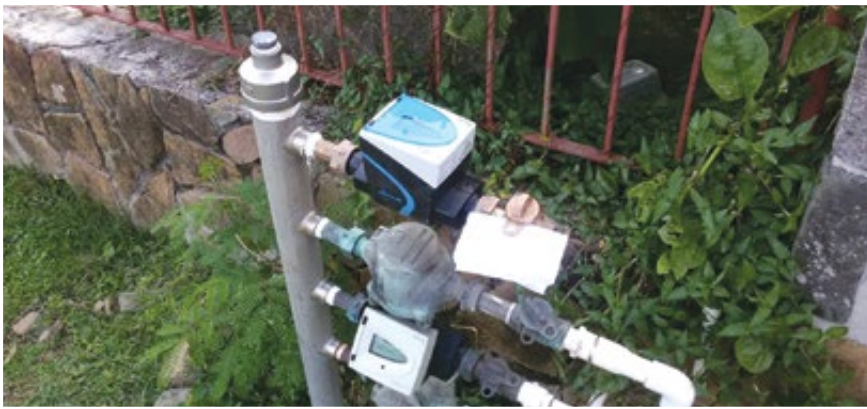
Newly installed water meter at St Peters Community Garden
